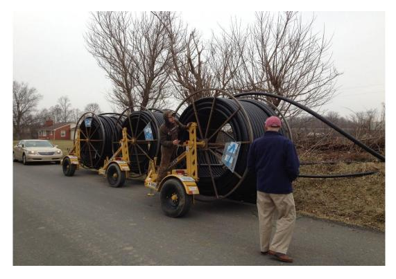
"Boring in the three conduit lines together for the 3-phase Delta 35kV system went smoothly with no installation issues. This allowed the project to be completed on time with no delays. By utilizing CIC, the labor savings eliminated any additional costs of pulling cable or any issue with excessive pulling tension on cable over the extended runs. The new power source was brought on line with no start up issues."
